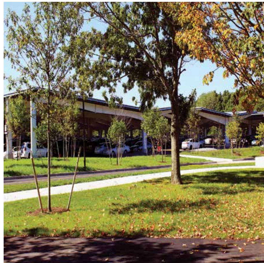
Solar canopy over lots 6-10.
