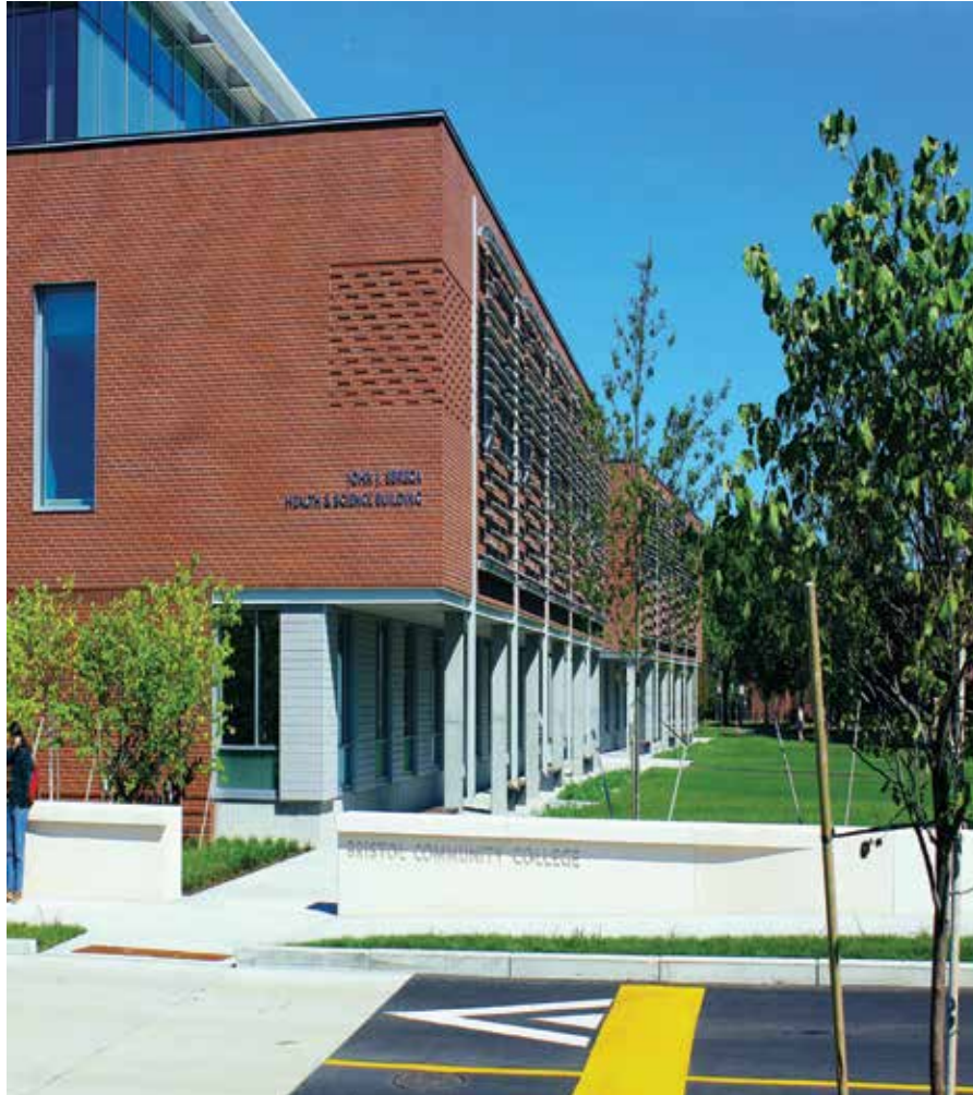
Side view of John J. Sbrega Health & Science Building.
