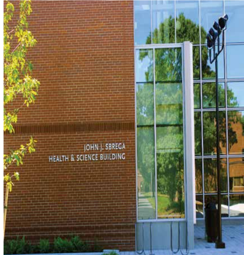
Front view of John J. Sbrega Health & Science Building.
